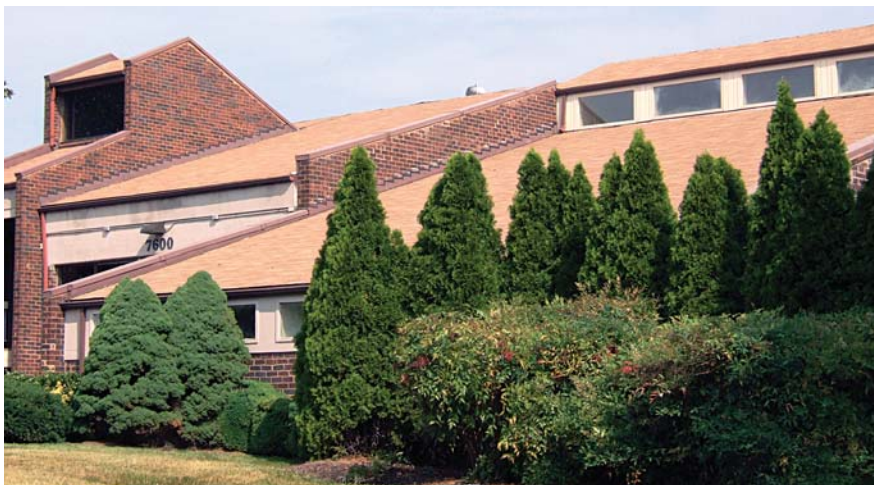
Greenbriar Community Building
